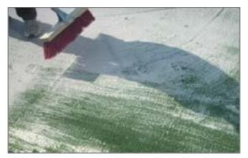
The infill of the artificial turf is a system in motion and the components of the infill move naturally during the game. This shifting is heightened in areas of more intense use. Periodical brushing is advisable to redistribute the sand.
