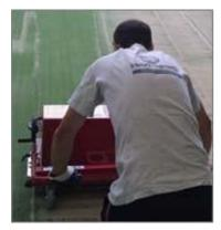
Silica sand infill can be unpacked and aerated using an apparatus equipped with a specific rotating brush that penetrates between the fibres of the artificial turf system.
