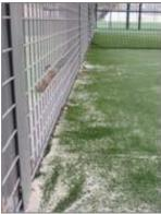
Irrigate the turf with water to clean the fibers and sand, and, at the same time, keep drainage holes clear and protect the court's sub-base drainage system.
